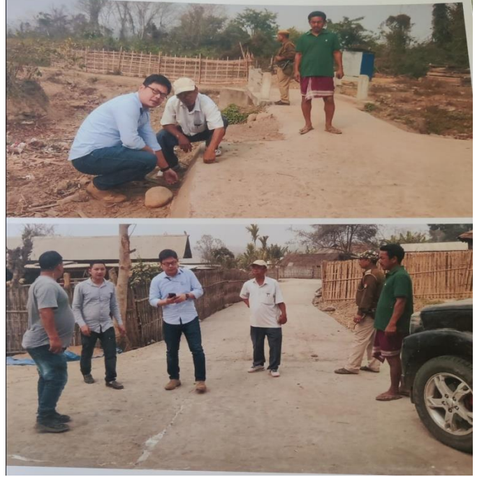
Name of work:-Construction of Cement Concrete Pavement at Prasadimdik Name of Scheme:-Axom Adarxo Gram Yojana 2019-2020
